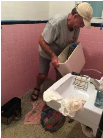
Erik Dalaker fixing the clogged toilet in the pink bathroom
